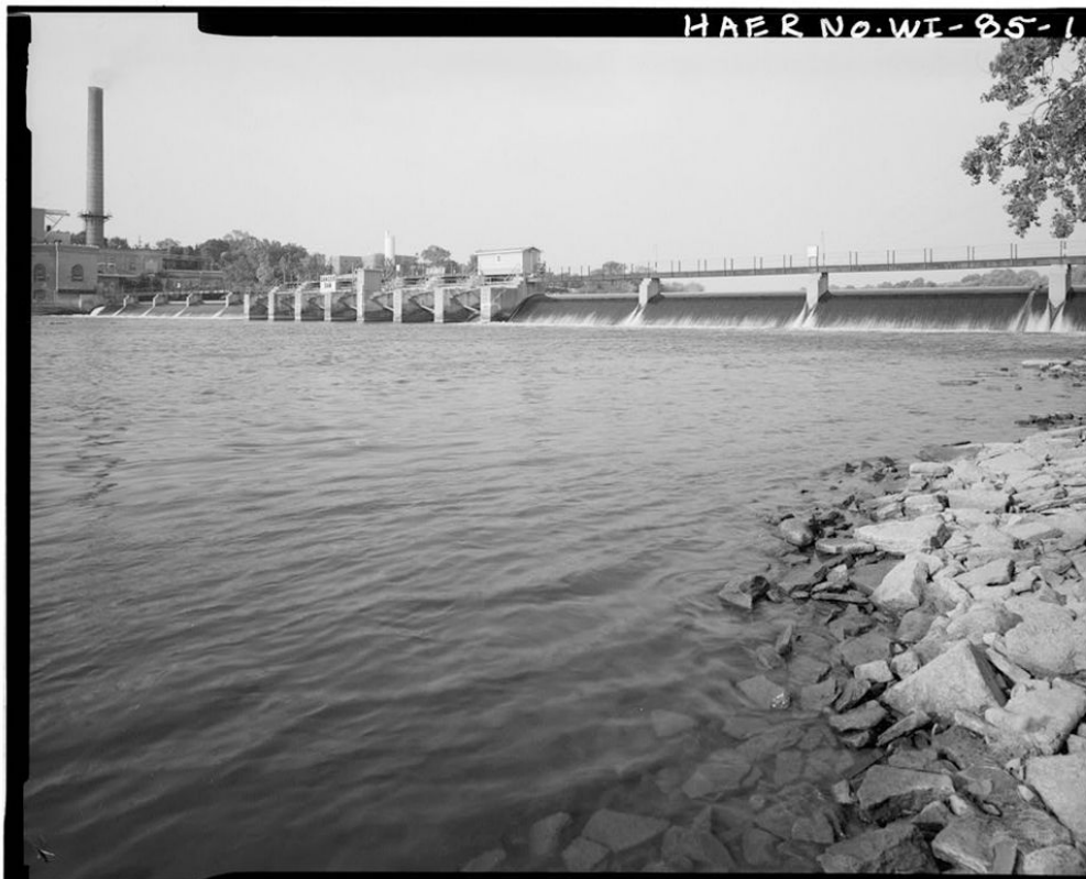
Figure 1: Fox River Dam, the first hydroelectric station built in 1882, in Wisconsin. PHOTOGRAPH FROM THE LIBRARY OF CONGRESS
