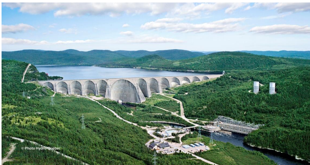
Daniel Johnson Dam and Manic-5 Generating Station on the Manicouagan River in Quebec (Source: Hydro-Quebec)
